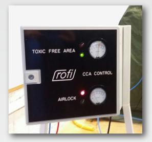
Pressure Indication Unit (PIU) shows the overpressure in each area and will alarm you visually if a pressure failure should occur to the system.
